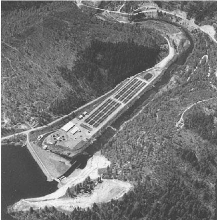
Aerial view of Lewiston Dam and Fish Hatchery on the Trinity River, built to mitigate loss of salmon and steelhead habitat associated with the construction of Trinity Dam. (Bureau of Reclamation)
