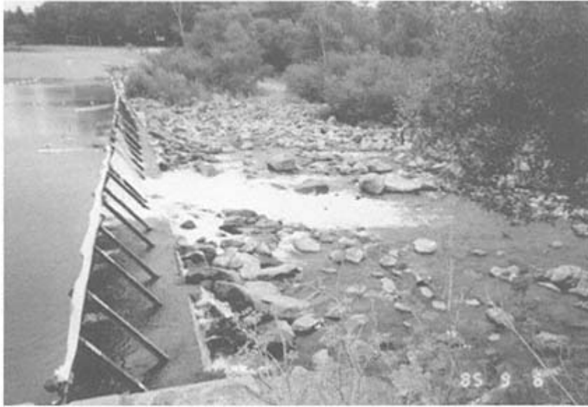
Seasonal dams with no fish protection facilities, like this one at Healdsburg, harm both upmigrant and downmigrant salmon and steelhead. (Stan Griffin)
