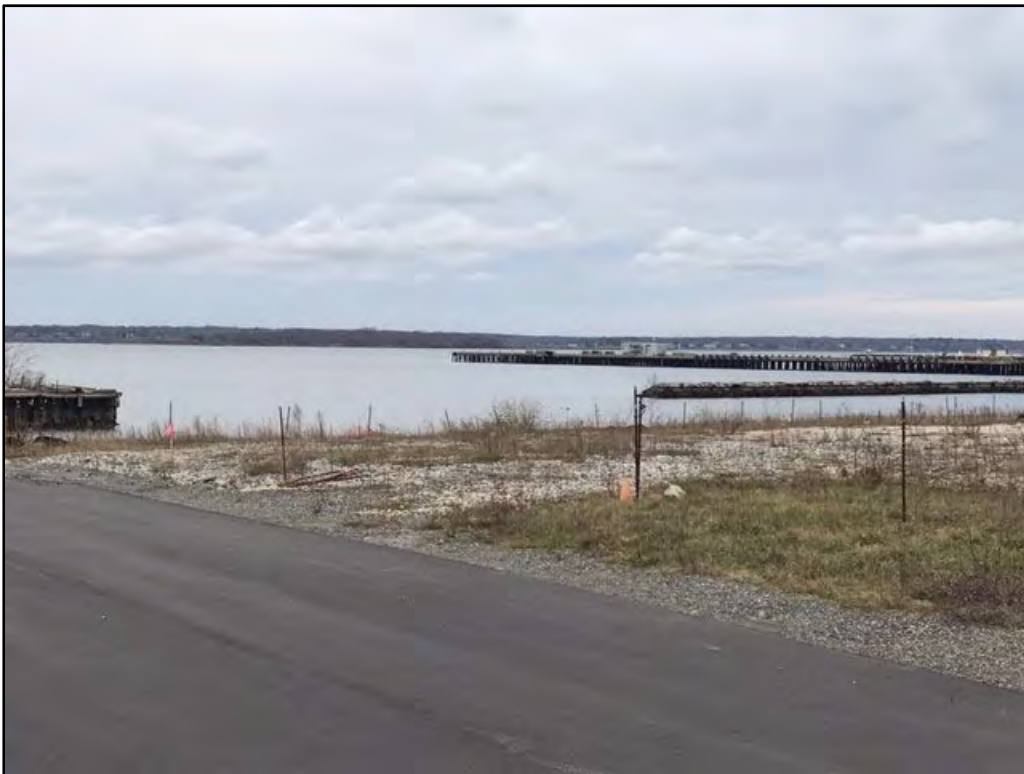
Photo 3. Pier Landing Site looking northwest towards Pier 2
