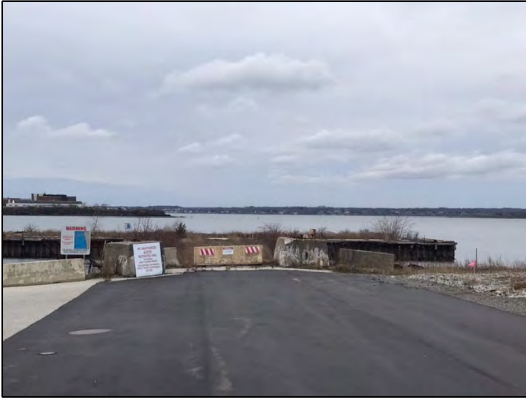
Photo 2. Pier Landing Site looking west towards T-pier
